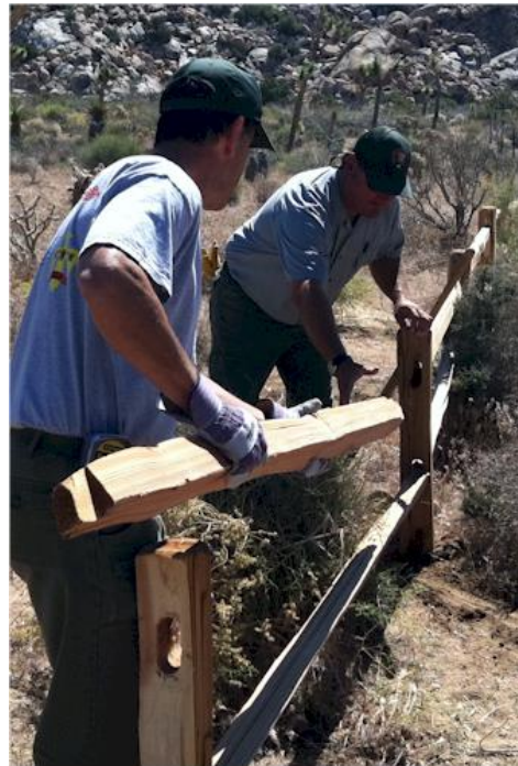
The OA hard at work replacing a split-rail fence in Joshua Tree. (Photo: M. Hare)
