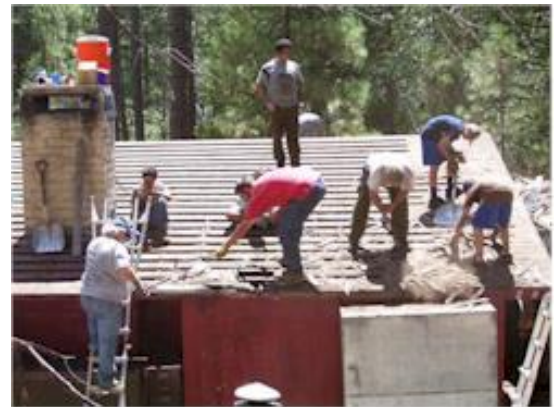
Members of Cahuilla Lodge work on a reroofing project on Boyce Lodge at Camp Emerson (Photo: S. McLeod)
